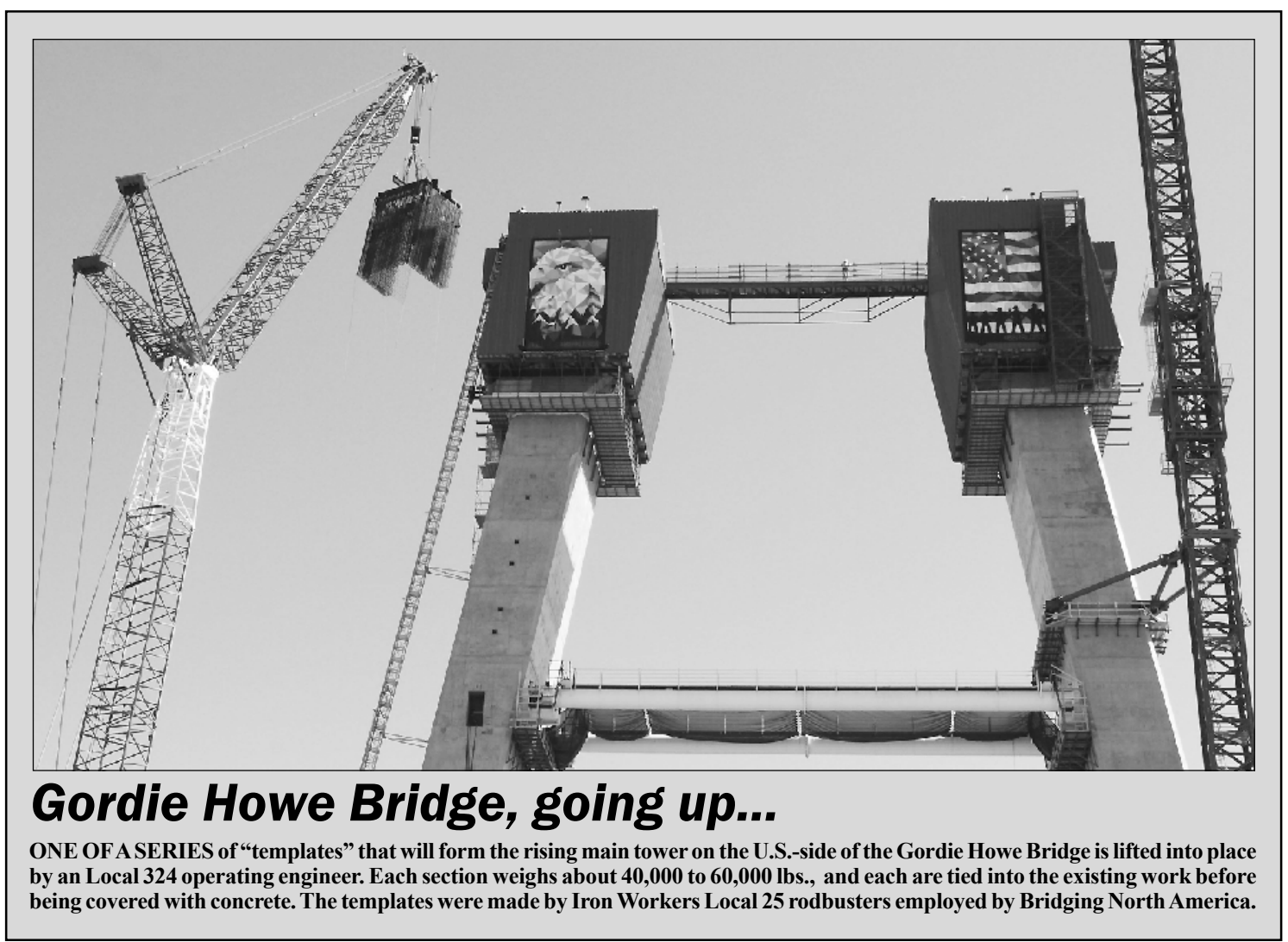
Gordie Howe Bridge, going up...
