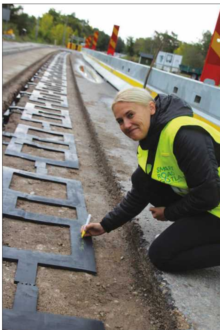
CHARGING COILS to wirelessly power electric vehicles are set in a road in Sweden prior to pouring the concrete by ElectReon, an Israeli company. Sweden also has a wired system. Photo credit: Electreon
