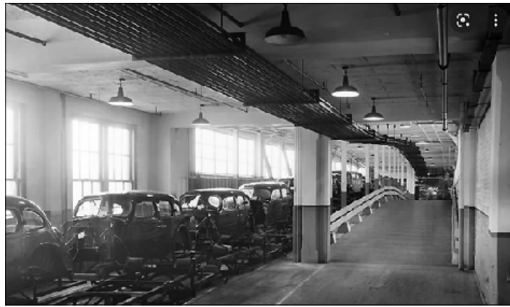
THE INTERIOR of the Packard plant, during production.
