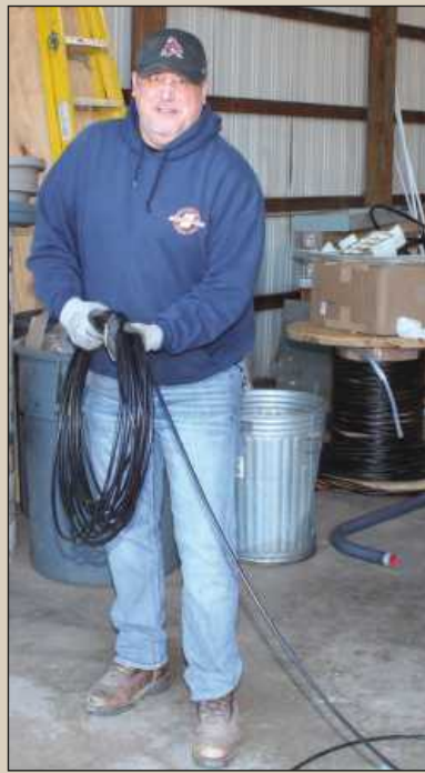
LOOPING CABLE for a generator at the Shouldice shop in Battle Creek is Ted Keaton, an IBEW Local 445 electrician.
