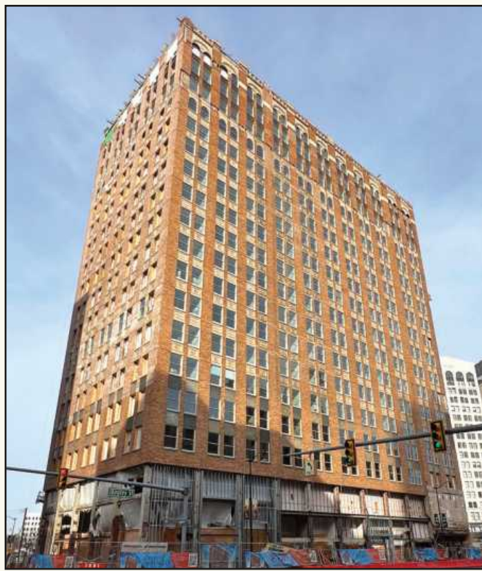
COMPLETED IN 1928, the former United Artists Building in Detroit was originally an office building. Today it's being converted into 148 apartments, the "Residences @ 150 Bagley." Abandoned in 1974 along with the demolished United Artists Theater that was in the rear of the building, the tower has now been empty longer than it was in use – but thankfully it remained in good condition structurally for redevelopment.
