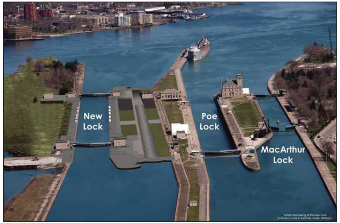
THE NEW LOCK at the Soo is nearly a decade-long project that will eliminate the existing Sabin and Davis locks, replacing them with a lock that will twin the size of the Poe Lock.
