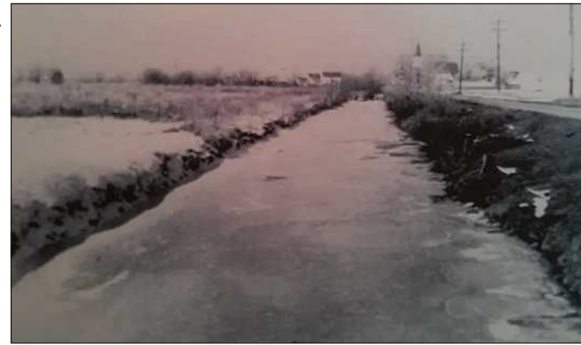
A SECTION OF THE CANAL looking west toward Hayes Road in Clinton Township, date unknown, likely early last century. Modern development have buried most of the original canal works. A towpath, at right, would allow for horses, oxen or mules to drag barges and other low-draft watercraft through the canal.
