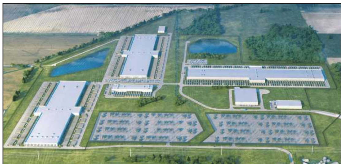
A RENDERING of the Stargate data center project in Saline Township.
