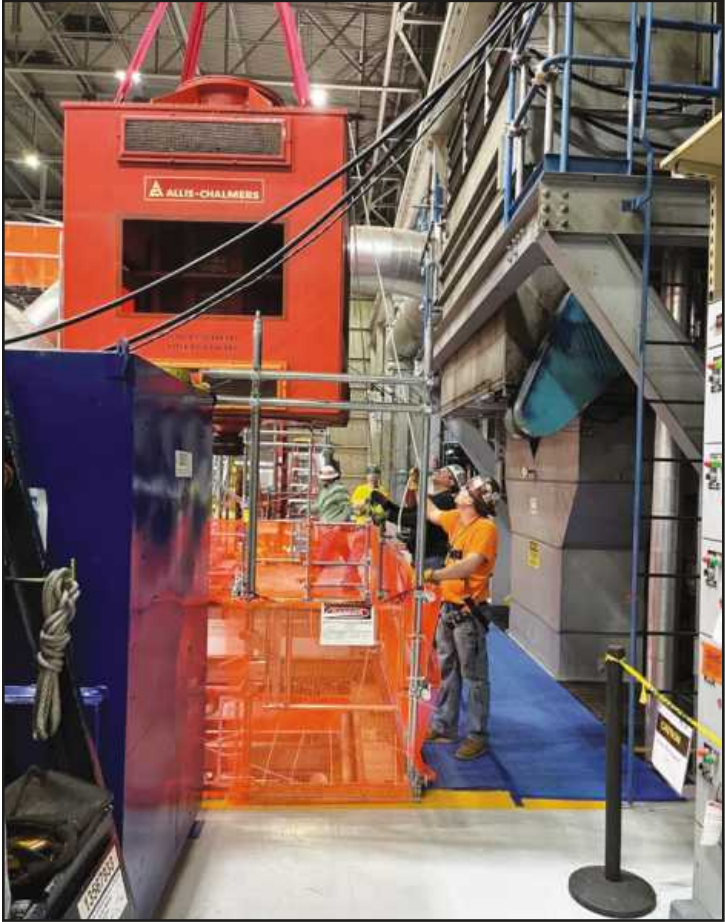
CONDENSATE PUMP motors are shown being removed for refurbishment last year from the Palisades Nuclear Power Plant.
