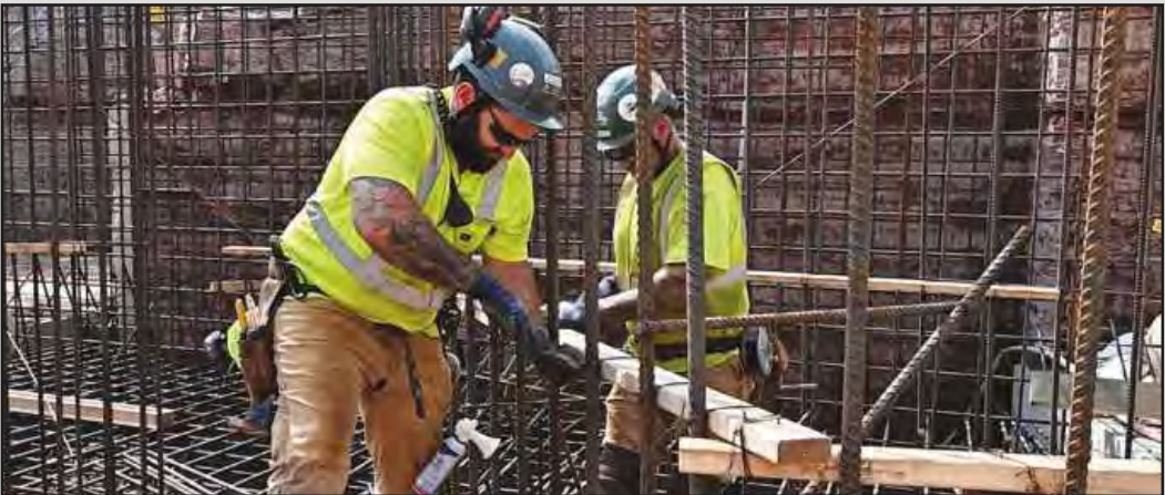
RODBUSTERS in Iron Workers Local 8's jurisdiction tie rod at the New Lock at the Soo project.
