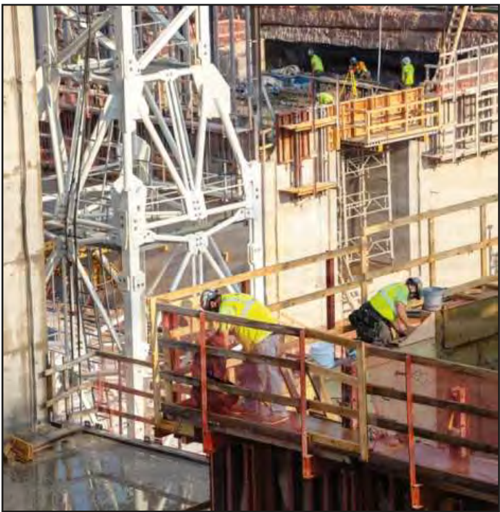
WORKERS WITH Kokosing Alberici Traylor prepare formwork on the New Lock at the Soo project in Sault Ste. Marie. The workers are setting the formwork for concrete monolith placements which creates the new lock chamber.
