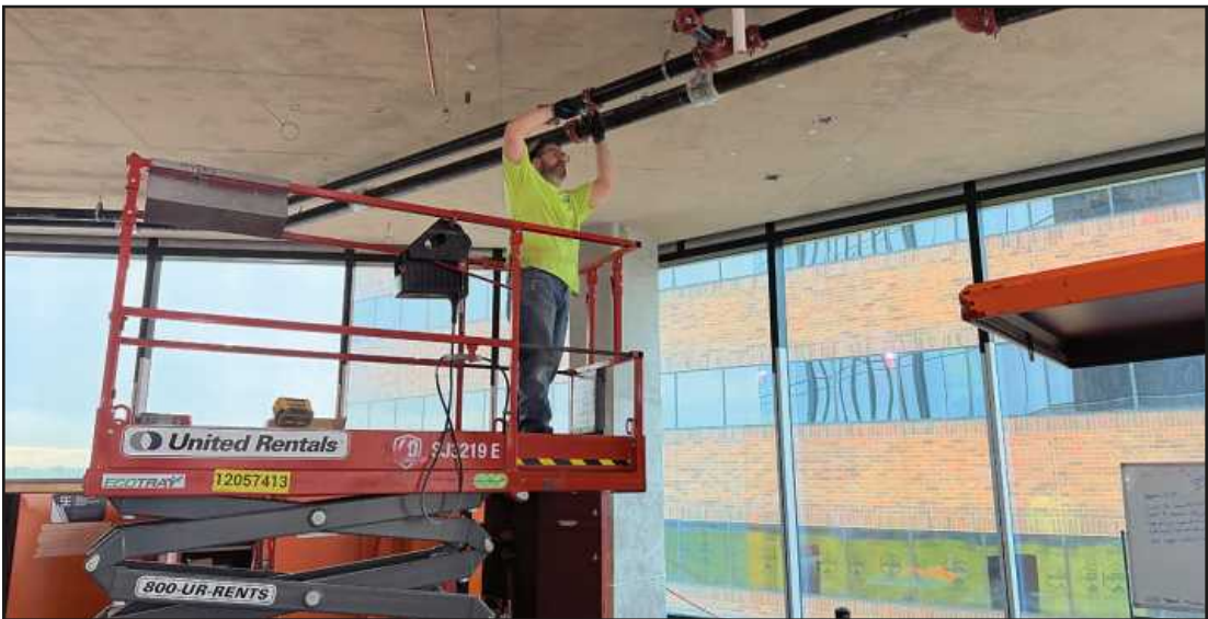
WORKING ON HEATING and cooling piping on the fifth floor of the New Vision tower project in Lansing is Scott Wilson of Plumbers and Pipe Fitters Local 333. He’s employed by Myers Plumbing and Heating. We will have more information and photos regarding this project in an upcoming edition.
