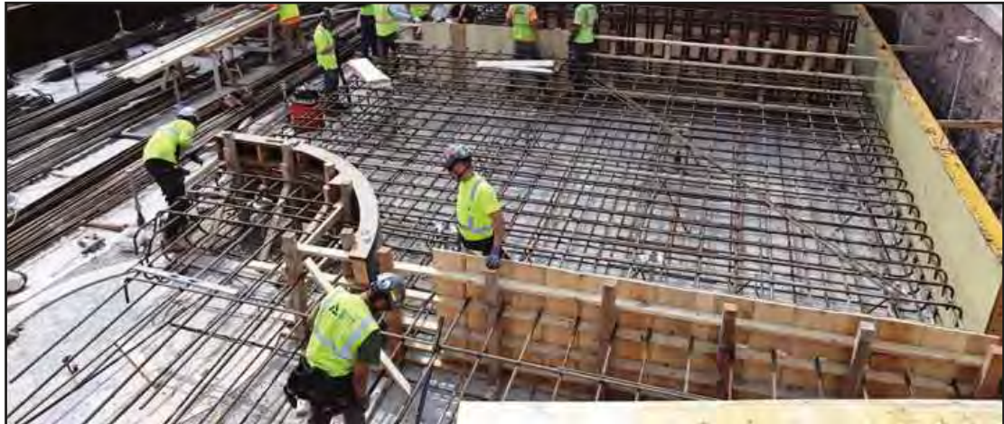
BUILDING TRADES WORKERS get ready for a concrete pour at the New Lock at the Soo project in Sault Ste. Marie.
