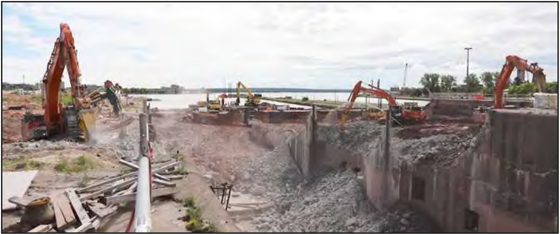
DEMOLITION OF THE Sabin Lock, which was completed in 1919, has been necessary in making way for the New Lock at the Soo.
