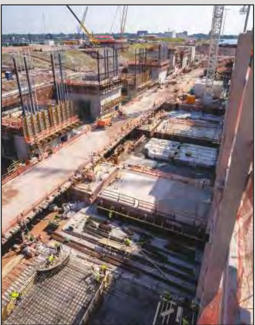
CONCRETE MONOLITHS take shape at the New Lock at the Soo project in Sault Ste. Marie. A total of 84 concrete monoliths — and a lot of rebar — will make up the new lock chamber, where 1,000-foot-long-plus freighters will traverse the locks.
