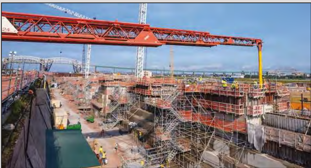
TRADES WORKERS with Kokosing Alberici Traylor place concrete to top off monolith S25 at the New Lock at the Soo project in Sault Ste. Marie. Each concrete placement is about five feet deep, and each monolith takes nine to 14 lifts to complete.
