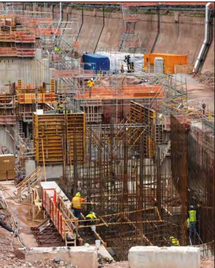
RE-BAR FOR CONCRETE monoliths take shape at the New Lock at the Soo project in Sault Ste. Marie.
