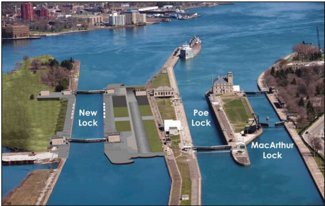
THIS IS AN ARTIST'S rendering of the completed New Lock at the Soo project. The new lock is being constructed in the footprint of the former Sabin Lock, and it will be the same size as the Poe Lock (completed in 1968, 1,200 feet long, 110 feet wide and 32 feet deep). The 800-foot-long MacArthur lock, at right, was completed in 1943. The locks are indispensable in allowing Great Lakes shipping to traverse the 21-foot drop in elevation at the St. Mary's River.
