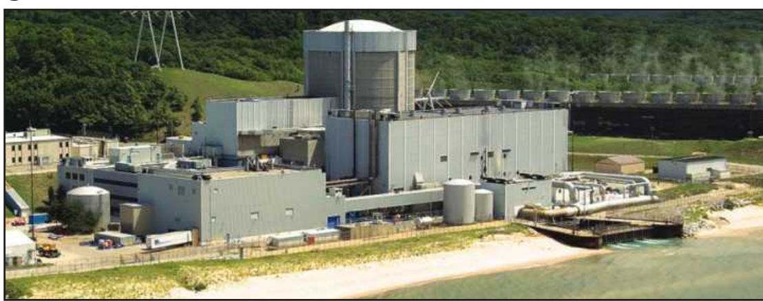
DELIVERY OF A FEDERAL loan of $1.52 billion will resurrect the Palisades Nuclear Power Plant, and the tasks ahead will employ hundreds of building trades union workers.
