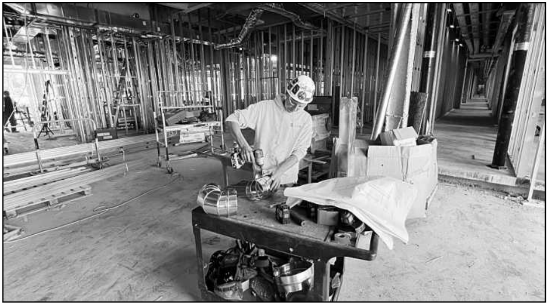
MAKING 45s - Brett Abbruzzese of Sheet-metal Workers Local 7 joins together duct elbows while working at the Lansing Public Safety building project.
