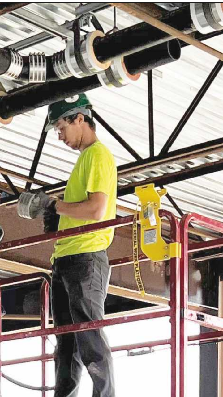
SETTING STORM DRAIN pipe while working at the Lansing Public Safety building project is third-year apprentice Shay Hiemstra of Plumbers and Pipe Fitters Local 333. He's employed by Johnson and Wood.
