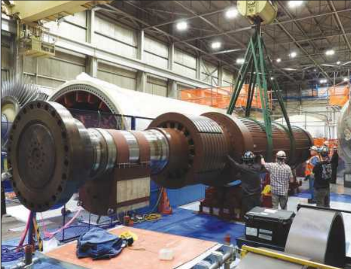
A 183-TON MAIN generator rotor is removed for inspection in Turbine Building at the Palisades Nuclear Power Plant. To date, The Building Tradesman has been unable to get access to the plant to take photos. Photo credits: Holtec
