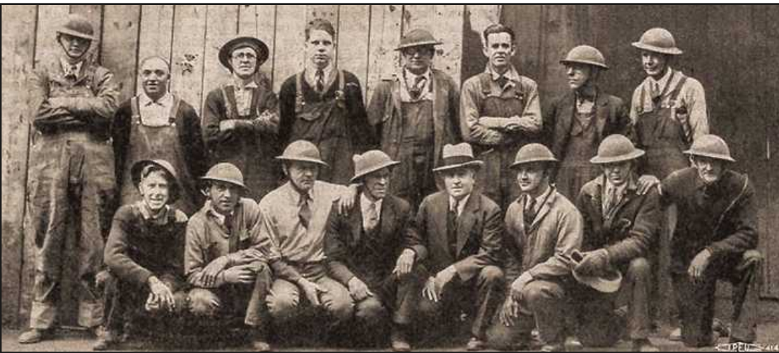
FALLING DEBRIS at a jobsite in Boston in 1931 spurred the IBEW innovation of using old World War I military helmets as head protection on construction sites.
