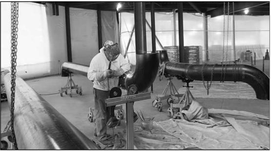
WELDING A 12-INCH CARBON STEEL hot water pipe at the State of Michigan public health and environmental science laboratory near Lansing is Josh Simon of Plumbers and Pipe Fitters Local 333. He's employed by John E. Green.
