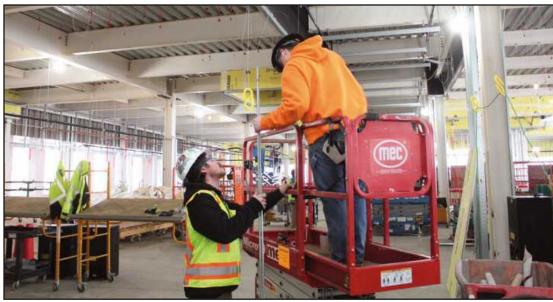
HANDING UP pipe hangers he cut at the State of Michigan public health and environmental science laboratory near Lansing is Tim Speagle of Plumbers and Pipe Fitters Local 370. On the lift is Justin Mulder of Plumbers and Pipe Fitters Local 333. They're employed by Gunthorpe Plumbing and Heating.
