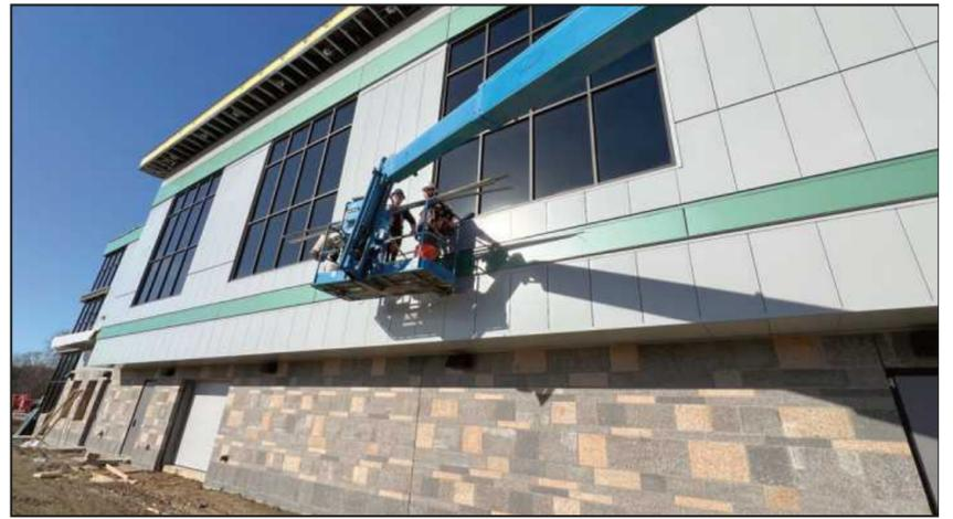
SETTING METAL PANELS on the new Berston Field House in Flint are Hunter Kuehn and Brandon Bancamp of Sheet Metal Workers Local 80. They're employed by Cass Sheet Metal.
