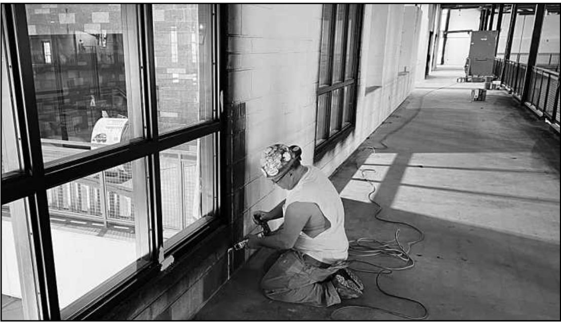
CAULKING A SEAM on the running track at the Berston Fieldhouse project in Flint is Rod Poley of Bricklayers and Allied Craftworkers Local 2. He's employed by HMC Mason Contractors.
