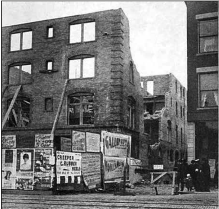
THE OTSEGO HOTEL IN Jackson after its concrete floors and a partial wall collapsed in 1902. The interior floors were rebuilt and the building opened in April 1904. Photo credit: Fireproof Magazine
