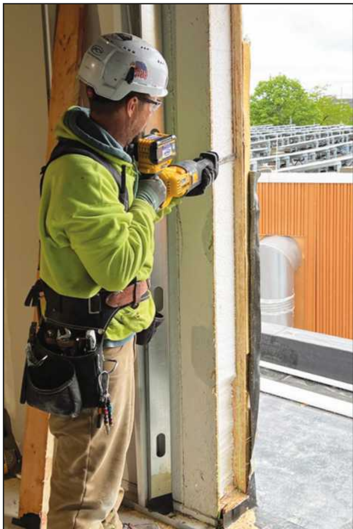
SLICING AN INSULATION panel as he prepares a frame for a door at the IBEW Local 58 expansion project in Detroit is Keegan Cole of Michigan Regional Carpenters Council Local 687. He's employed by Pontiac Ceiling and Partition.
