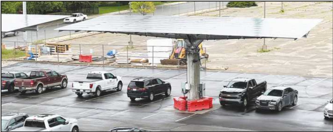
SOLAR TRACKING panels that tilt to follow the sun offer a super-efficient way to collect energy. Three of these 35x60-foot panels are set in the parking lot of IBEW Local 58.
