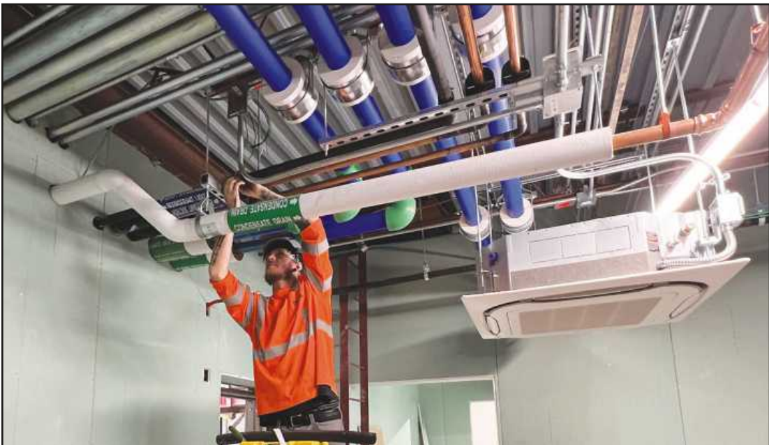
INSULATING A REFRIGERANT line in what will be kitchen space at the IBEW Local 58 union hall expansion in Detroit is Jacob Huff of Heat and Frost Insulators Local 25. He's employed by Rival Insulation.
