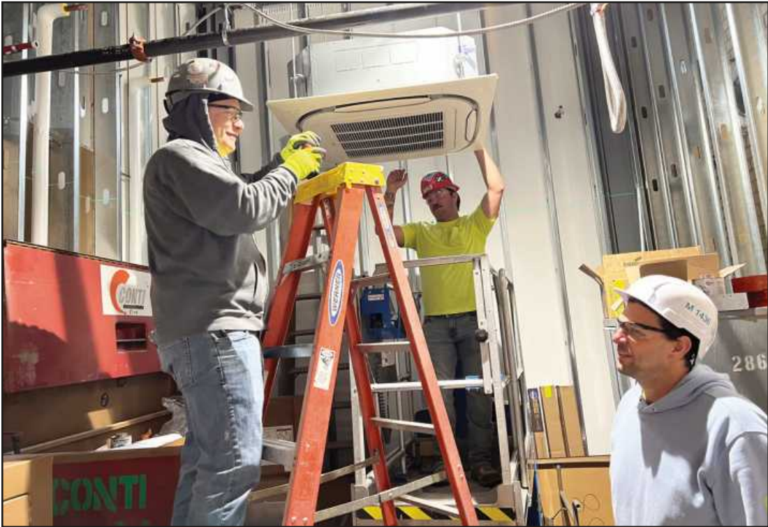
A TRIO OF PIPE FITTERS set a VRF cassette used in the heating and cooling system of the addition to the IBEW Local 58 union hall in Detroit. The Local 636 members include Dan Stuckey, Scott Haugh and Kevin Locher. They’re employed by Conti.
