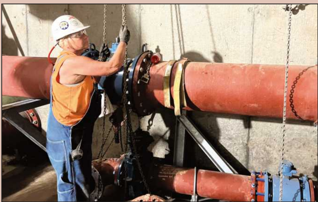
SETTING A NEW 16-inch discharge pipe at the Saline Wastewater Treatment Plant is foreman Lori Joseph of Plumbers and Pipe Fitters Local 190. She's employed by J.F. Cavanaugh Co.
