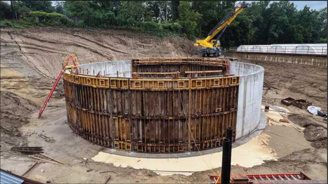
A SECONDARY CLARIFIER, a tank that uses gravity to separate solid particles (like sludge and scum) from wastewater. is shown under construction at the Saline Wastewater Treatment Plant.
