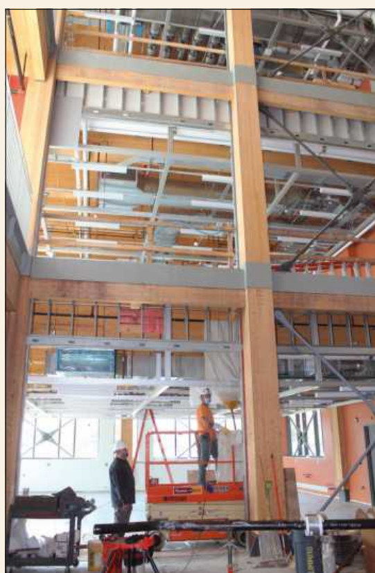
AT WORK IN THE south annex of the STEM project at Michigan State University are (l-r) Ken Stevenson and Jeremiah Ramsey of Plumbers and Pipe Fitters Local 333. They're employed by Gunthorpe, working near a lattice of engineered, exposed, old-growth timber that will add a tremendous amount of character to interior.
