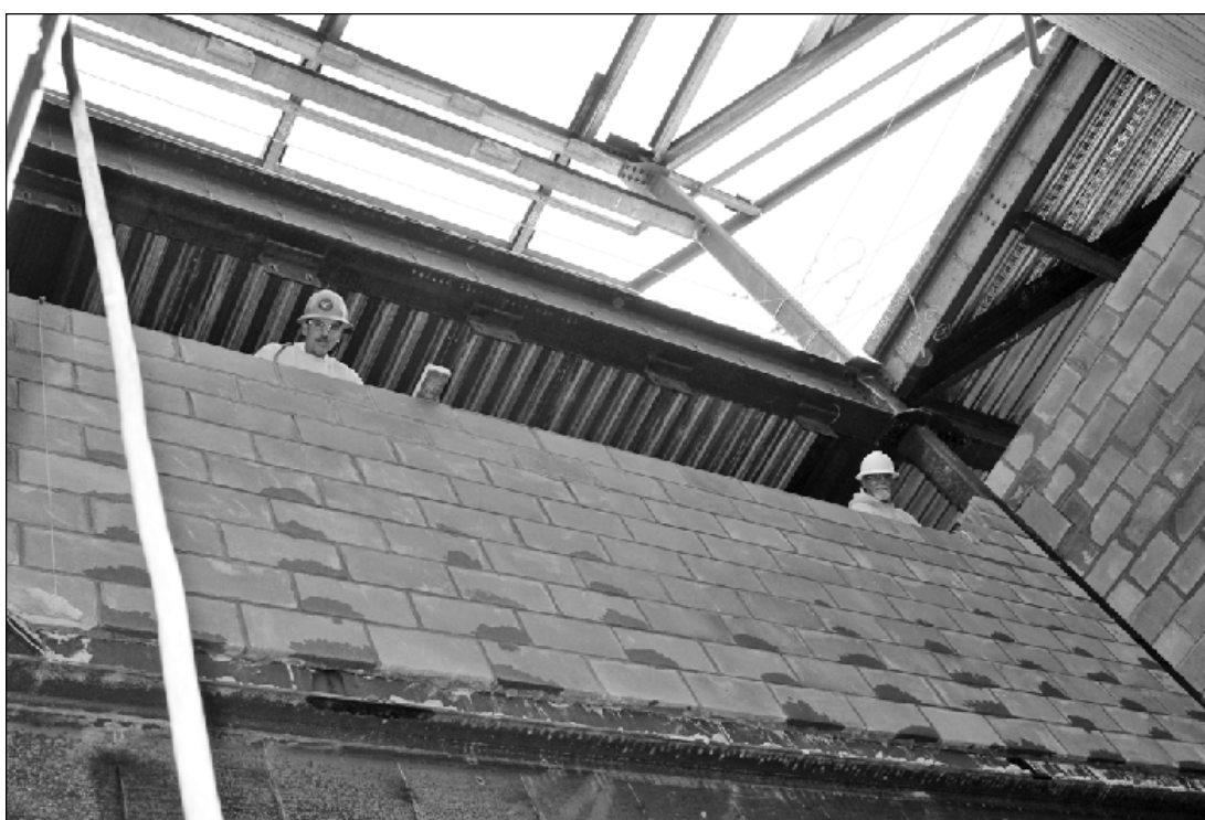
MASONS Joe Young and Chuck Labeau of Bricklayers and Allied Craftworkers Local 2 build an interior block wall at the Owosso Memorial Hospital project. They're employed by Davenport Masonry.
