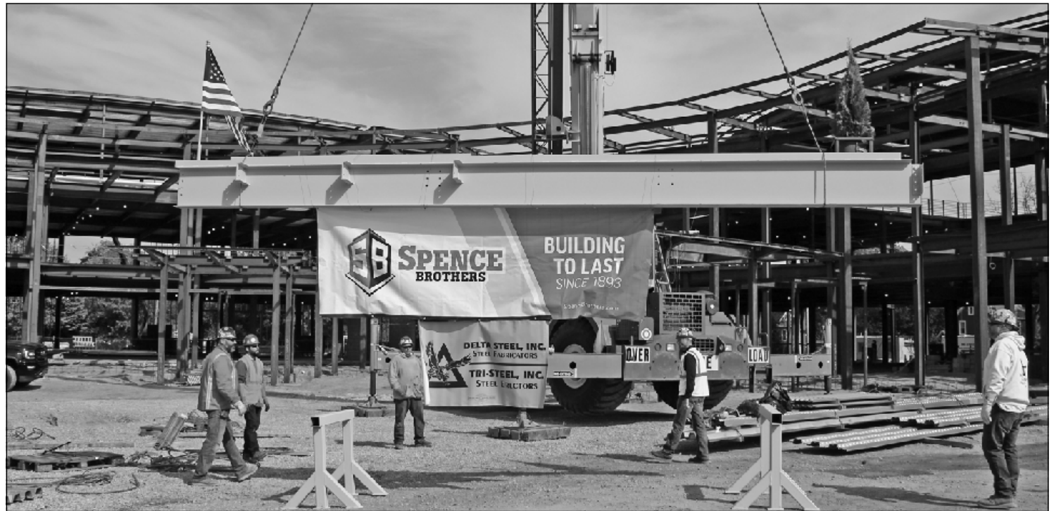
LOCAL 25 IRON WORKERS and a Local 324 Operating Engineer raise the final structural section of steel this month on the Owosso Health Care’s new neurological and orthopedic and wellness center. Spence Brothers is managing the project, while Tri-Steel handled the steel erection and Delta Steel did the fabrication.
