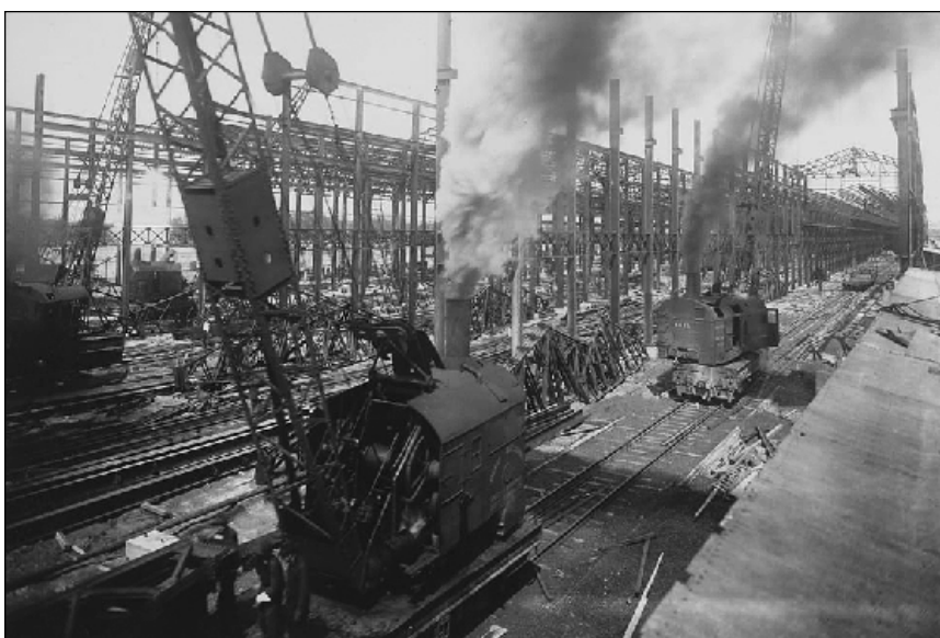
CONSTRUCTION OF the Ford Rouge plant was in full swing in May 1918.
