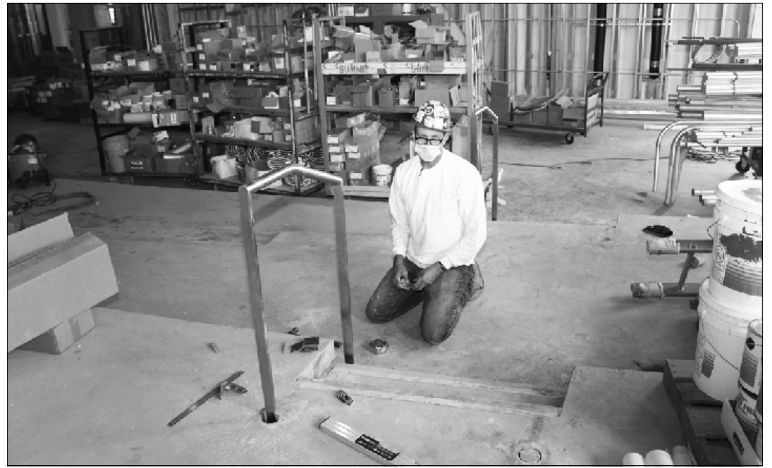
INSTALLING A HAND RAIL in a classroom at the Michigan State University STEM project in East Lansing is Jeff Rosier of Iron Workers Local 25. He's employed by Couturier Iron Craft.
