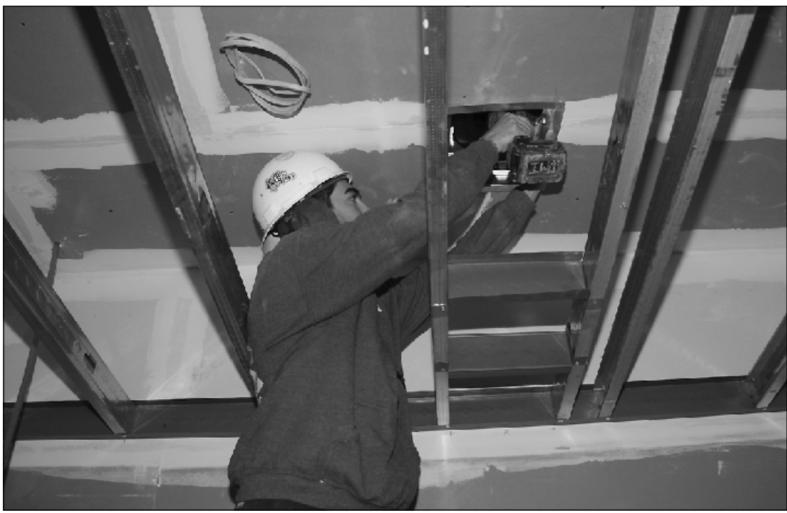
SETTING DUCT WORK at the Beacon House project in Marquette is Noah Brooks Sheet Metal Worker Local 7. He's employed by DMI. Photo by Jack Deo
