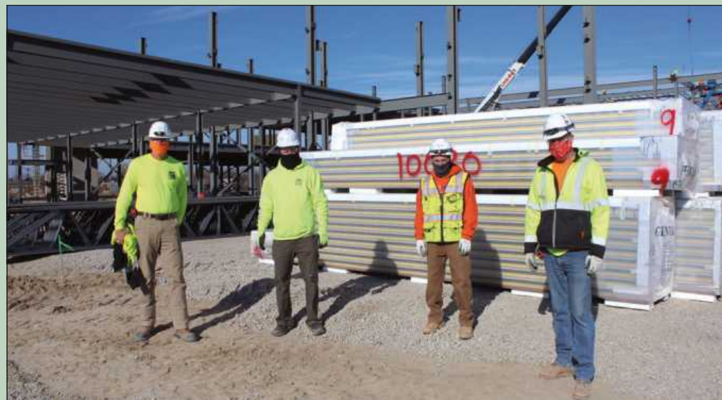
PAUSING FOR A PHOTO in front of the new Michigan Regional Council of Carpenters and Millwrights building they're helping to erect are a group of MRCC Local 687 journeyman Carpenters. They include (l-r) Mike Wisusik, Joe Decker, Vince Morandi and Troy Cameron. They're employed by Christman Constructors.
