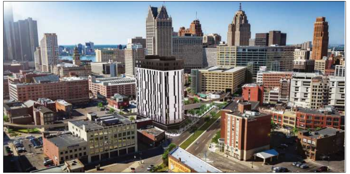
A RENDERING OF the 16-story Exchange Building that’s currently going up in Detroit’s Greektown. It will have a mix of apartment and condominium units. Under a plan by Barton Malow and the LiftBuild system, individual floors will be built on the ground and lifted into place.
