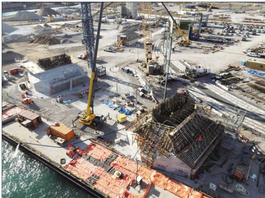
CONSTRUCTION OF THE Gordie Howe Bridge will be simplified, somewhat, by a design that keeps the piers out of the Detroit River. Image credit: Bridging North America
