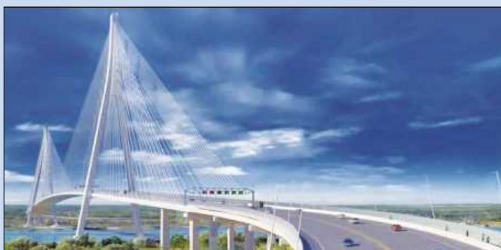
A RENDERING of the Gordie Howe International Bridge over the Detroit River, which will be of a cable-stay design — much cheaper to build with precast concrete than a steel-heavy suspension design like the nearby Ambassador Bridge. This will be the longest cable-stay span in North America.
