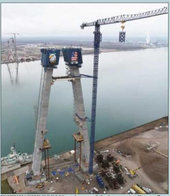
WITHIN THE FORMS at the top of the legs, according to Construction Connect, concrete is poured through rebar, with a total of about 130 cubic yards for a typical "lift" or segment. The forms then "climb" to the next level through a series of support (Continued on Page 2) brackets and screw jacks, powered by electric motors.
