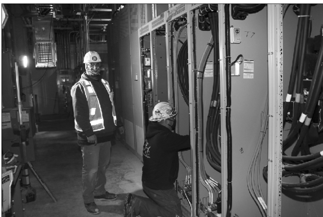
AT WORK CABLING A 480-volt panel at the Lansing Board of Water and Light's Delta Energy Park plant are (l-r) Jeremy Soli of IBEW Local 665 and Greg Anderson of IBEW Local 58. They're employed by Superior/Motor City Electric.
