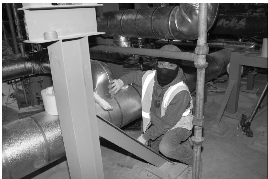
SEALING A DUCT at the Lansing Board of Water’s new Delta Energy Park powerhouse is Brennan Dunham of Heat and Frost Insulators Local 47. He’s employed by Advance Industrial Services.
