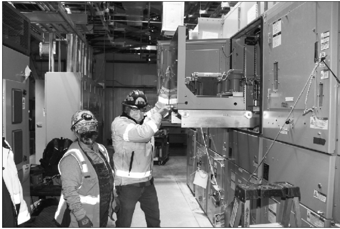
ELECTRICIANS (l-r) Carrie Talbor and Carl Sander of IBEW Local 665 pull out a breaker on a 4160 volt panel at the Lansing Board of Water and Light Delta Energy Park power plant. They're employed by Superior/Motor City Electric.
