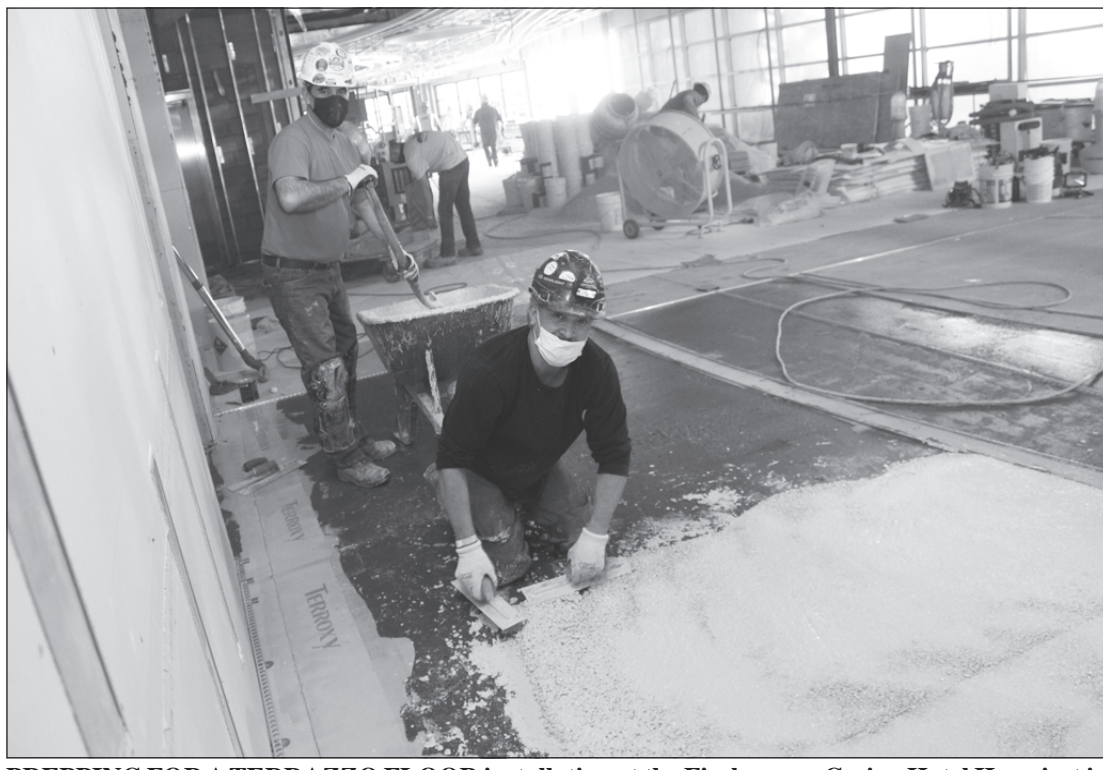
PREPPING FOR A TERRAZZO FLOOR installation at the Firekeepers Casino Hotel II project in Battle Creek are Miguel Franco and Ruben Gallegos of Bricklayers and Allied Craftworkers Local 2. They're employed by Artisan Tile.
