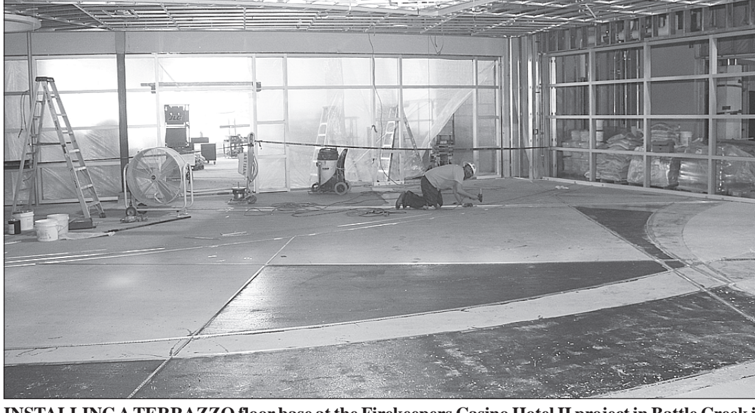
INSTALLING A TERRAZZO floor base at the Firekeepers Casino Hotel II project in Battle Creek is Rodney Gillean of Bricklayers and Allied Craftworkers Local 2. He's employed by Artisan Tile.
