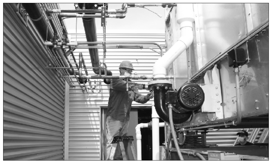
INSTALLING HEAT TRACE on a cooling tower at the expansion project at Battle Creeks Kellogg Airport is Marty Preston of Plumbers & Pipe Fitters Local 333. He's employed by Mall City Mechanical.
