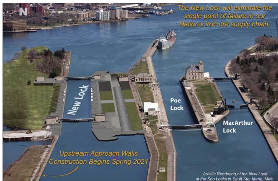
THIS IMAGE is a rendition that illustrates the completion of a second Poe-sized lock at Sault Ste. Marie. The new lock will replace two of the smaller, older locks on the left. The Poe Lock, which opened in 1969, was the last lock built in the Soo Locks system, and is the only passage between Lake Superior and the lower lakes capable moving the larger bulk freighters on the Great Lakes.
