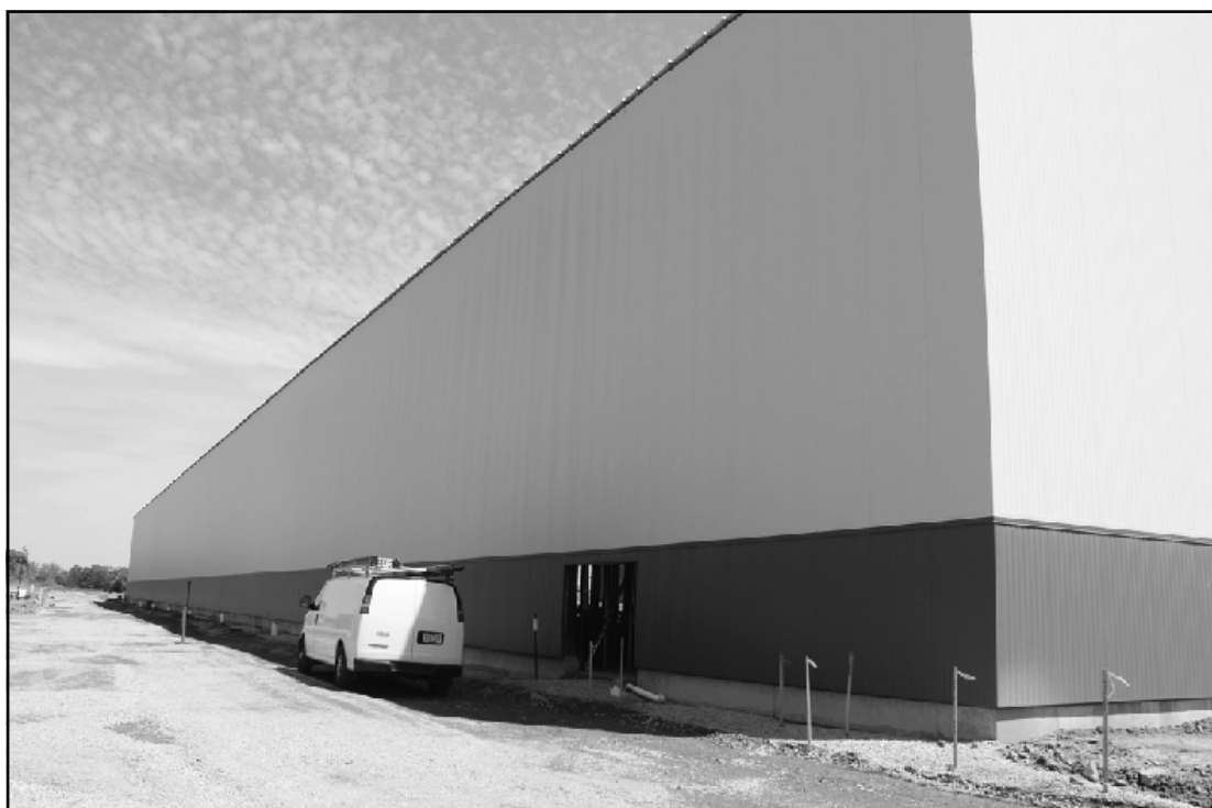
THE DAKKOTA-KETTERING project on Detroit's east side has been described as a "Big Costco," with 300,000 square-feet of space under 39-foot-tall metal walls on a six-inch concrete pad. The project will create 625 jobs for the automotive supplier. The $55 million project is currently employing about 90 tradespeople, working under project manager Devon Industrial Group.
