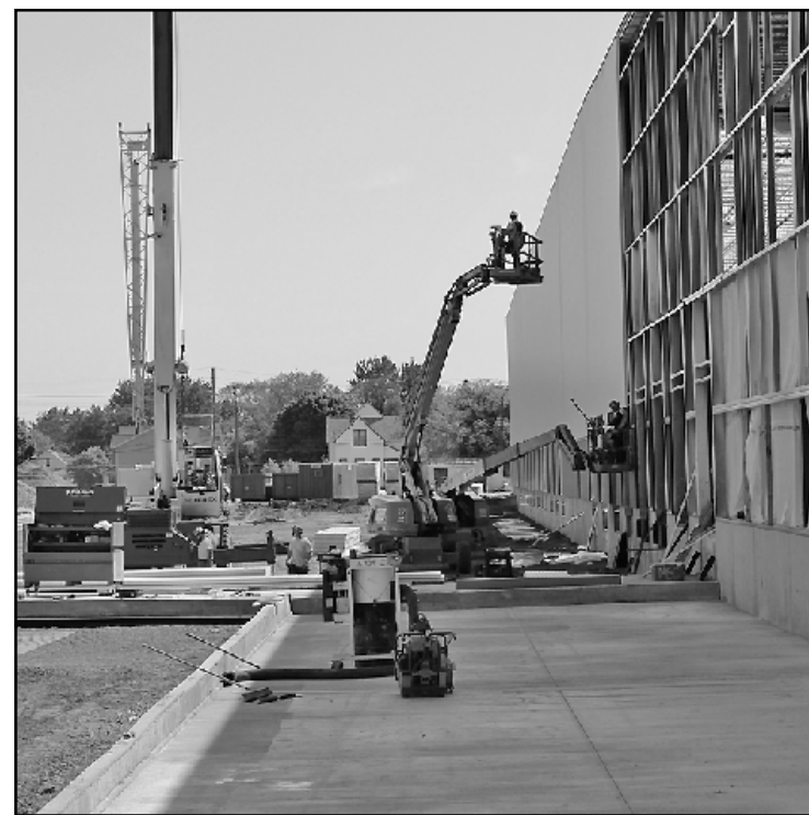
READYING A CURB for a cement pour by installing expansion paper are Local 1076 Laborer Tyler Denski and Local 687 carpenter Karl Smith. They're employed by Devon Industrial Group at the Dakkota-Kettering project in Detroit.
