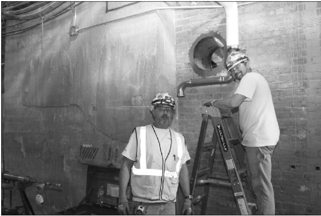
RUNNING THREE-INCH copper lines for the use of the domestic water system at the Ford-Michigan Central Station in Detroit are Joe Rorick and Tony Szalkiewicz of Plumbers Local 98. They're employed by W. J. O'Neil.
