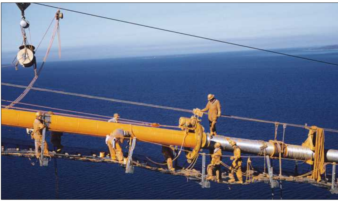
MACKINAC BRIDGE PAINTERS wear some of the orange primer they're applying on a main cable near the top of the South Tower, on Oct. 4, 1957. The bridge opened to traffic on Nov. 1, 1957. Modern inspections have shown the main cables in nearly pristine condition due to the proper application of that paint and subsequent coatings over the years. Photo credit: MDOT
