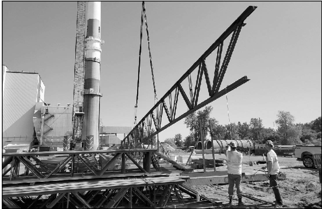
LOCAL 25 IRON WORKERS employed by Redinger Steel start to set a 140-foot truss while working at the Lansing Board of Water and Light's new Delta Energy Park. Photo credit: Marc Crance
