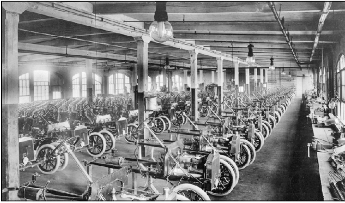
HENRY FORD'S new Piquette Avenue Plant in Detroit, 1904. The plant was among the last auto manufacturing plants to be built using wooden floors on timber framing – but it did have several fireproofing features, including sprinklers and fire doors. The four edges of each vertical post were also chamfered, so that their edges won't burn so quickly in the event of a fire. Photo credit: The Henry Ford
