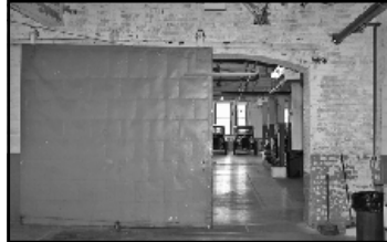
LARGE STEEL fire-proof doors at the Piquette Plant seal off one building section from another in case of fire.
