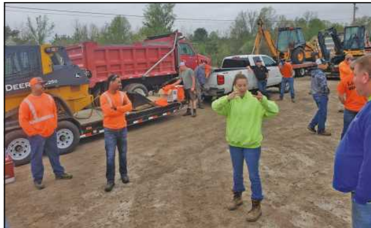
VOLUNTEERS affiliated with the Michigan Laborers Training and Apprenticeship Institute brought in much-needed heavy equipment on Memorial Day weekend to help clear debris in the Sanford area following the flood.
