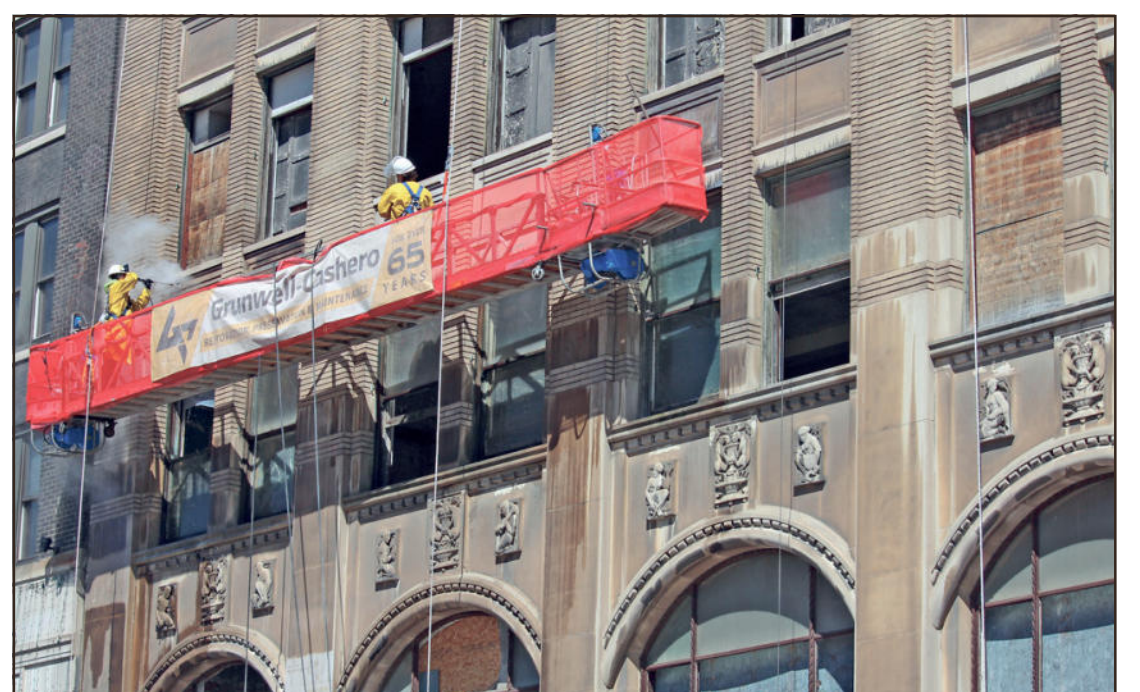
POWER-WASHING the 98-year-old brick and limestone exterior of the Park Avenue Building in Detroit are Laborer Rudy Leon and mason Tyler Tabor of Bricklayers and Allied Craftworkers Local 2. They're employed by Grunwell Cashero. The derelict building is getting readied for renovation after being empty since the 1990s.
