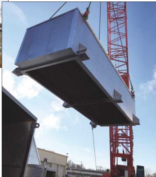
UNLOADING A SECTION of the the economizer at the Graphics Packaging project in Kalamazoo is work done by Capital City Crane's Local 324 operator and Boilermakers working for Barton Malow Co.
