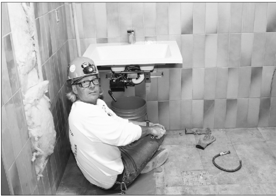
PLUMBER Joe Brooks of Local 98 sets a supply line for a second-story lavatory sink while working at the Michigan Carpenters Training Center in Detroit. He's employed by John E. Green.
