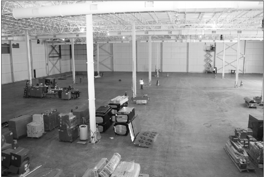
THE HIGH-BAY AREA for training at the Michigan Regional Carpenters Council Training Center under construction in Detroit.
