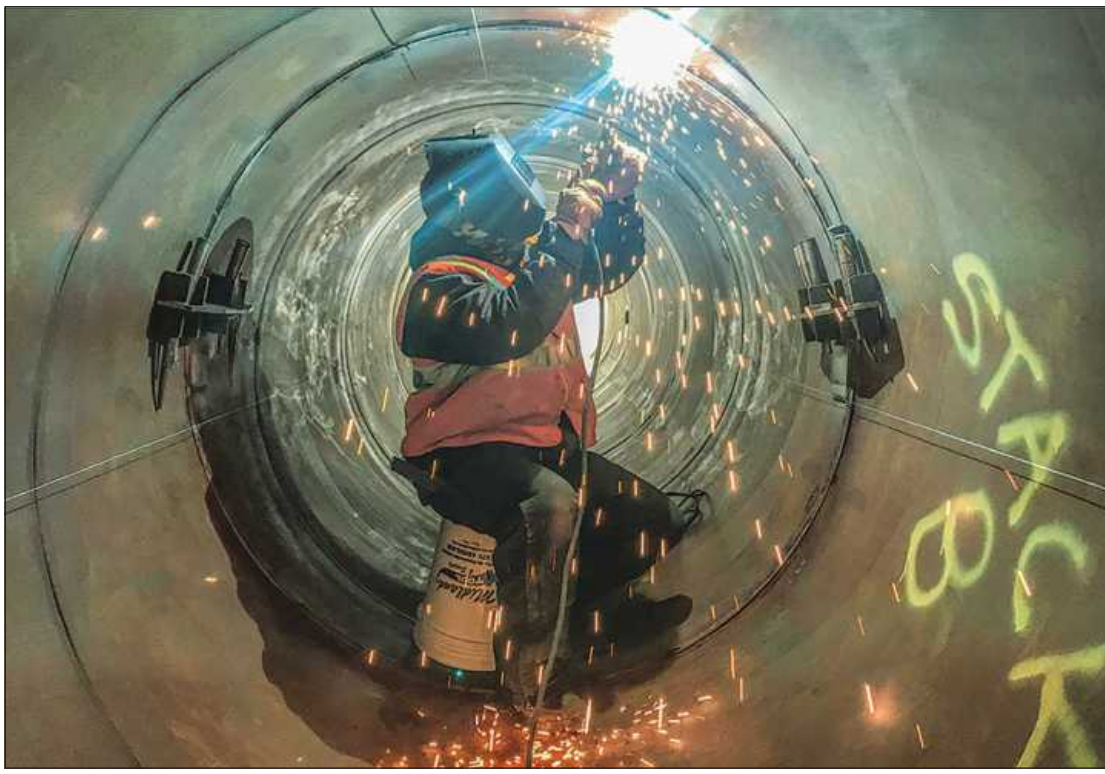
AT THE GRAPHICS PACKAGING expansion project in Kalamazoo, welding stack sections together is Boilermakers Local 169 member Sean Mckellip. He's employed by Barton Malow.
