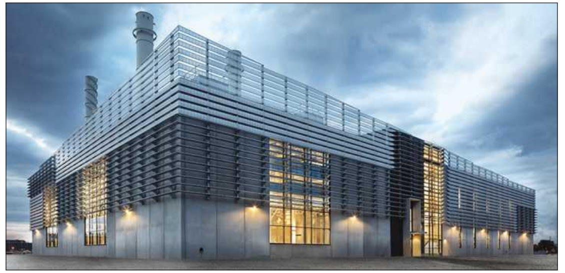
THE 35-MEGAWATT natural gas fuel-ed co-generation plant in Dearborn, owned by DTE Energy for use on Ford's Dearborn campus, was named Union Project of the Year by the Association of Union Contractors.
