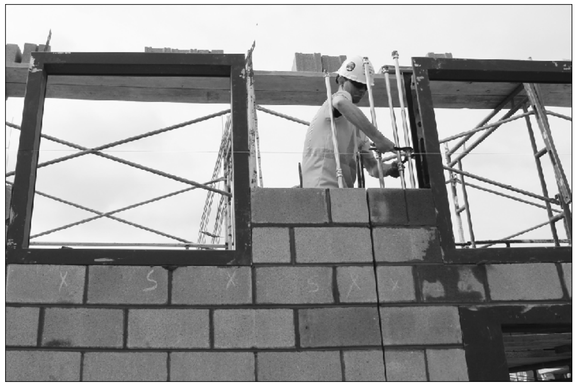
JOINING CONDUIT sections in a cell wall of the new Genesee County Juvenile Detention Facility is Aden Williams of IBEW Local 948. He's employed by Superior Electric.
