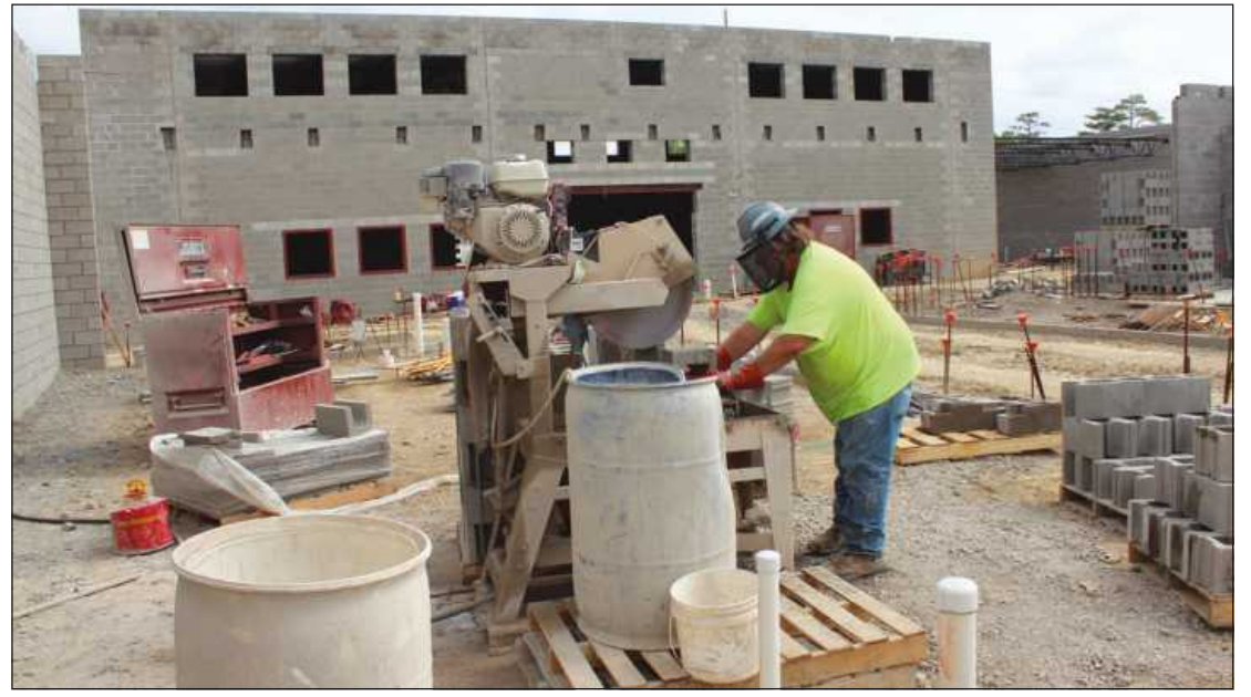
CUTTING BLOCK – lots and lots of block – at the Genesee County Juvenile Detention Facility project in Flint Twp. is Wayne Franklin of Bricklayers and Allied Craftworkers Local 2. He's employed by Davenport Masonry. The masons are the primary craft on the project, building numerous cell, interior and exterior walls.
