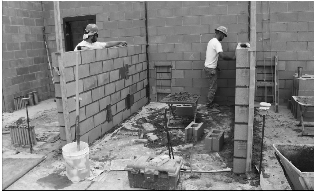
LAYING BLOCK walls that will be cell walls at the Genesee County Juvenile Detention Facility in Flint Twp. are (l-r) Christopher Cordeiro and Jordan Zimmer of Bricklayers and Allied Craftworkers Local 2. They're employed by Davenport Masonry.
