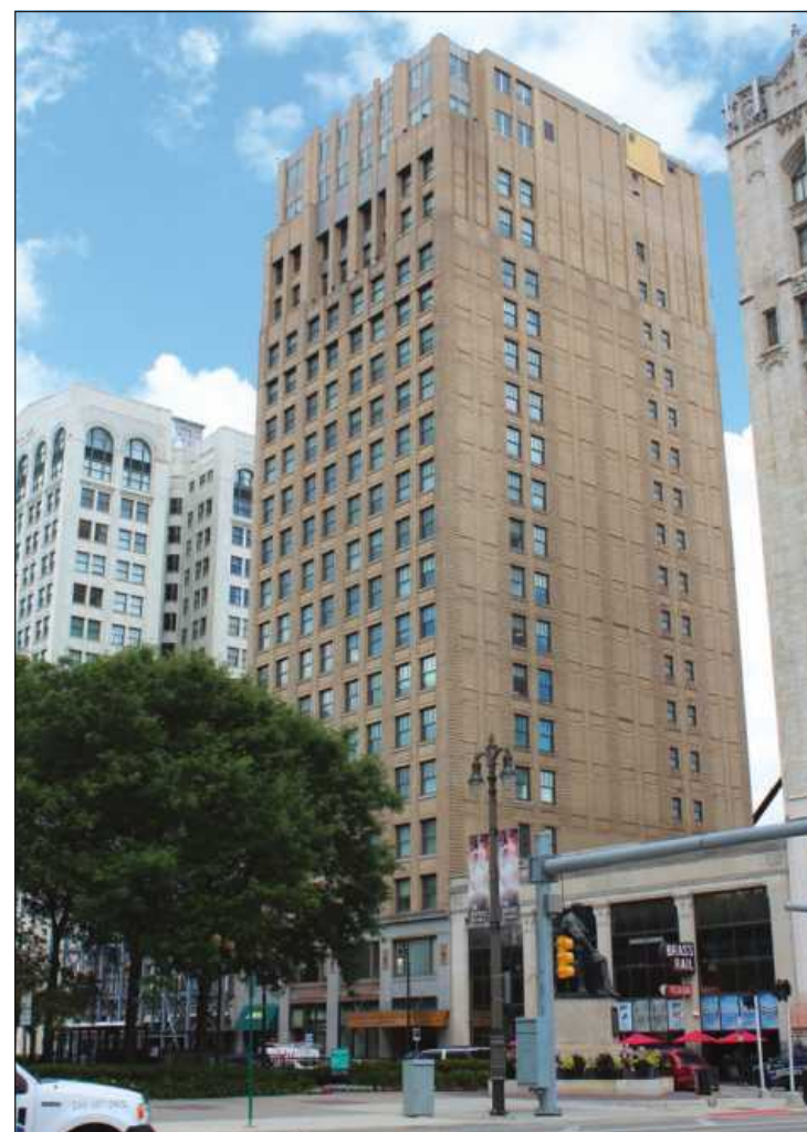
ERECTED AT A COST OF $2.5 million in 1921 for the Stroh Co., the 250-foot-tall building in Detroit is now known as Grand Park Centre. It's exterior masonry is undergoing rehabilitation.
