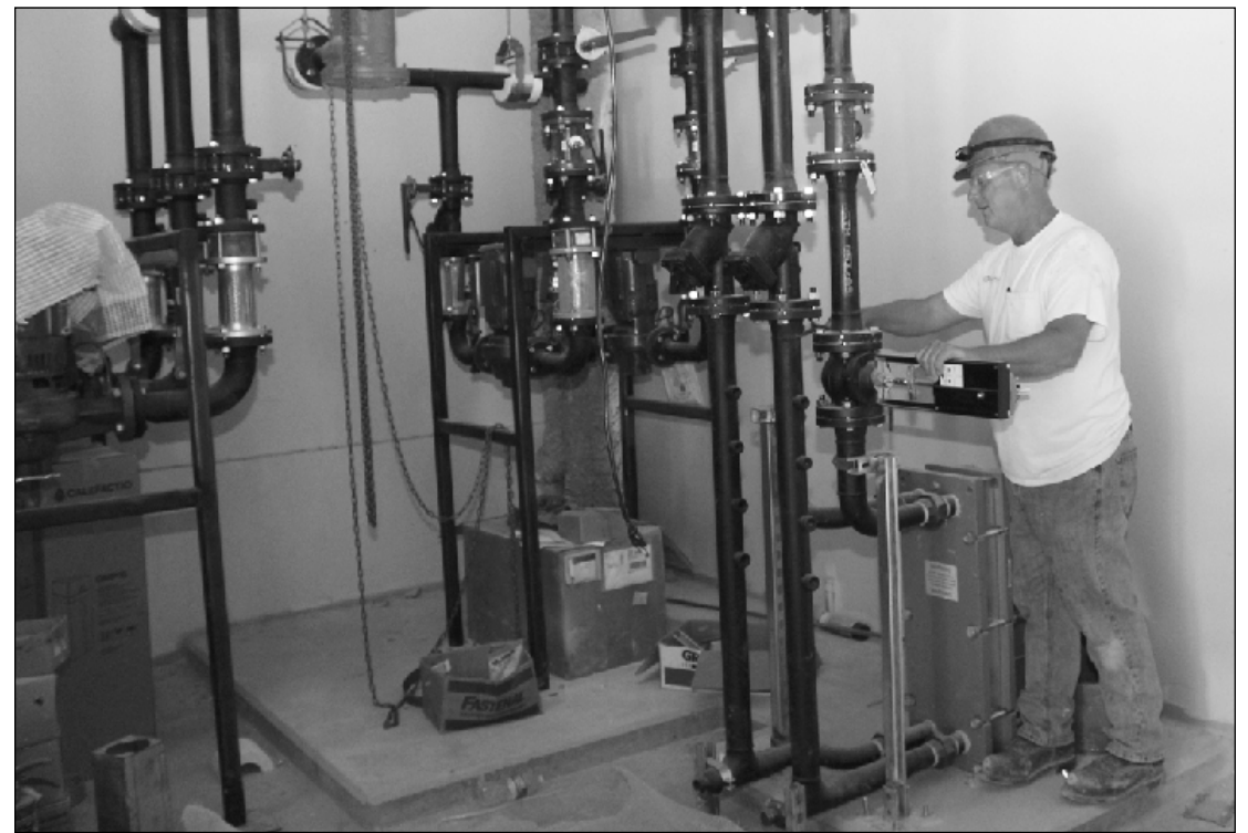
AT WORK ON THE BOILER/PUMP/HEAT EXCHANGER system on the first floor of the Mary Free Bed project at Covenant Health Care in Saginaw is Jerry Moore of Plumbers and Steamfitters Local 85. He's employed by Johnson and Wood.
