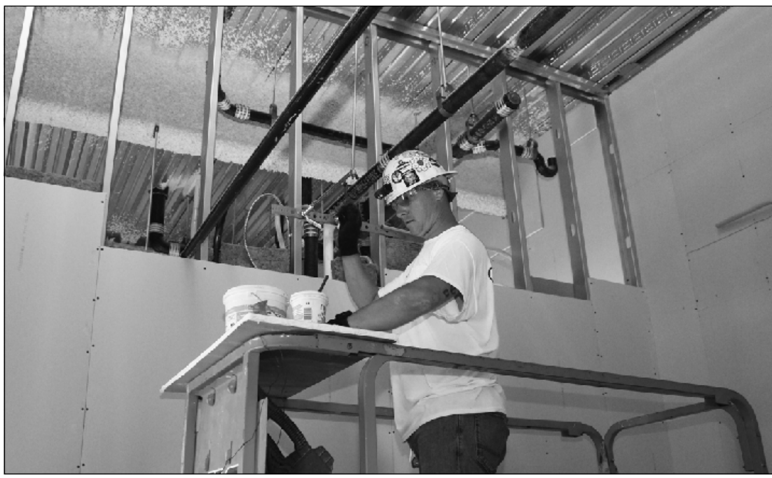
SETTING A 1/2-INCH WATER LINE in the upper reaches of a first floor patient exam room of the Mary Free Bed project in Saginaw is fifth-year apprentice Josh Musinski. The Plumbers and Steamfitters Local 85 member is employed by Johnson and Wood.
