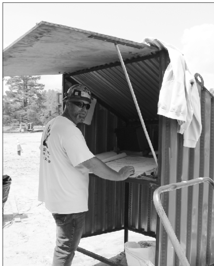
MADE IN THE SHADE: checking plans at the Caro State Psychiatric Hospital project is Tri-Steel foreman Dave Nelson of Iron Workers Local 25.
