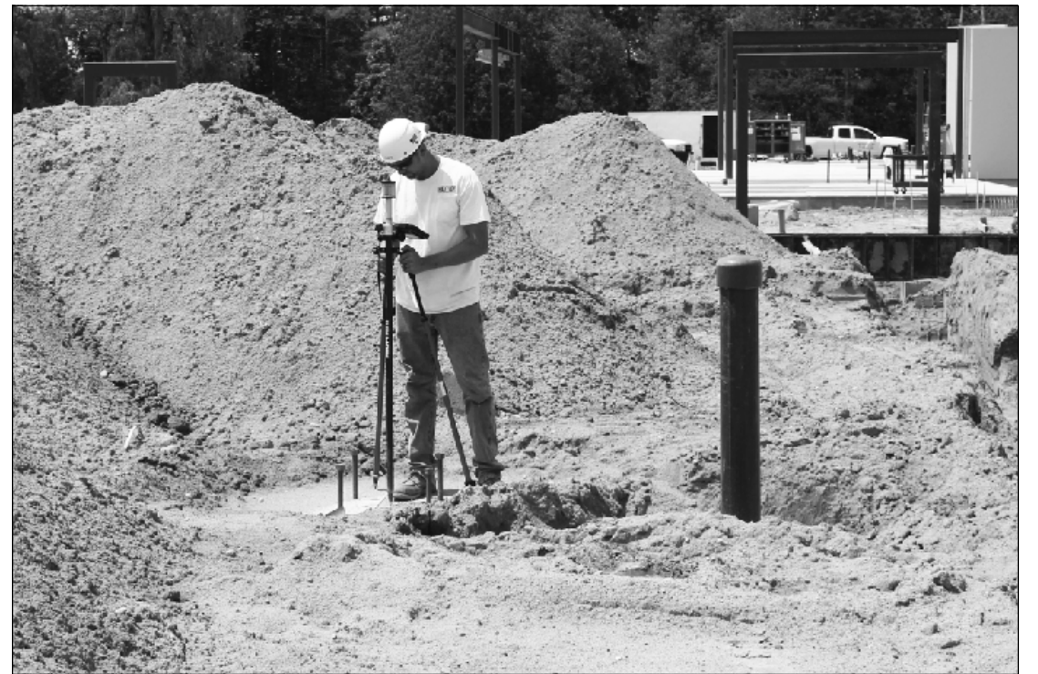
PEERING THROUGH A "Hilti Layout Tool" that aids plumbers with pipe placement is foreman Clint Claypool of Plumbers and Steamfitters Local 85. Employed by Remer, he's working at the Caro Psychiatric Hospital project.
