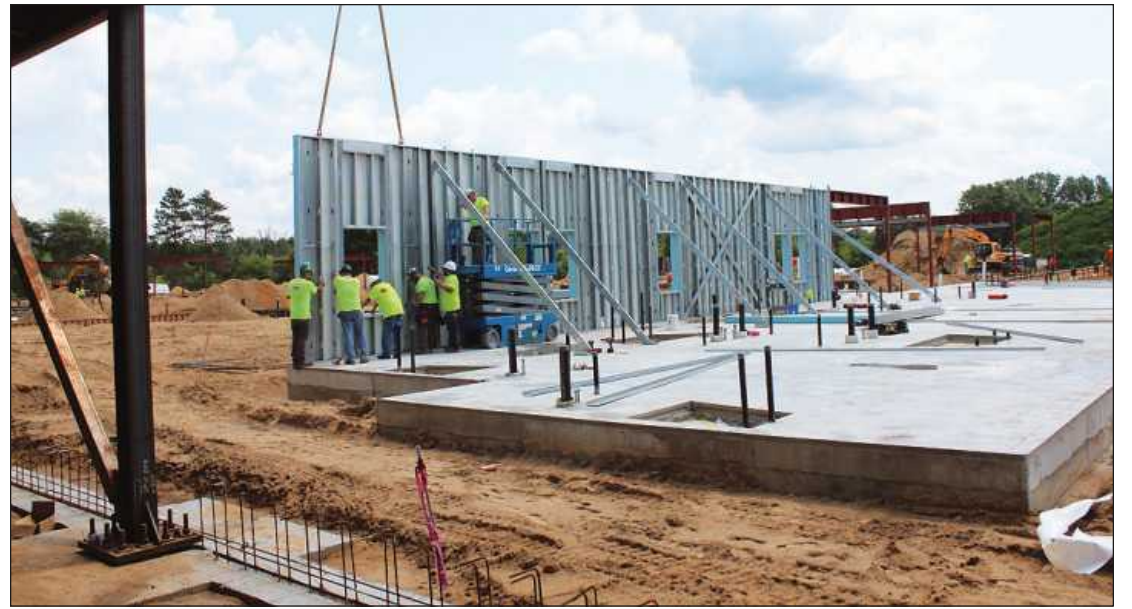
A GANG OF CARPENTERS sets up a prefabricated wall on the western side of the Caro Psychiatric Hospital project. They're employed by Accoustical Arts.
