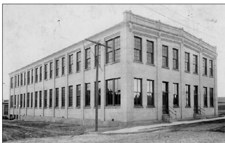
THIS IS THE FIRST AC Spark Plug building, shown in 1909 on Industrial Avenue in Flint. Photo credit: Buick City Blogspot
