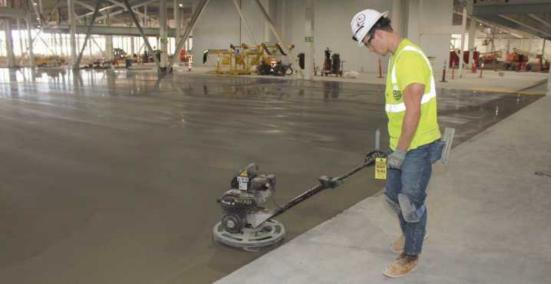
SMOOTH OPERATOR: Finishing part of the 2.8 million square-feet of floor at the Ultium Cells battery plant under construction in Lansing is Jeremy Pilch of Bricklayers and Allied Craftworkers Local 2. He's employed by Barton Malow.
