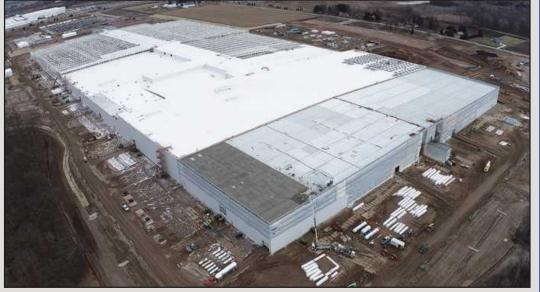
AT 2.8 MILLION SQUARE FEET, THE Ultium Cells plant under construction in Lansing along I-69 near I-96 is about s large as they come in Michigan. Currently it's mostly a shell inside, but in the coming months more than 1,000 building trades workers will be on site, installing hardhare and systems to build electric-vehicle batteries. The project is a joint venture of LG **Energy Solution and General Motors.**
